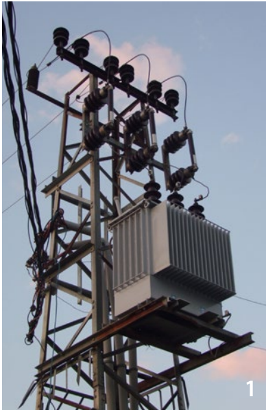
1 Transformatormasten aus Stahlgitter mit Stützisolatoren 10-20 kV (Noshpal ID315) – Totfund Weißstorch C. ciconia – 1 Transformer pole made of steel mesh with pin insulators, 10-20 kV (Noshpal ID315) – found dead White stork C. ciconia
