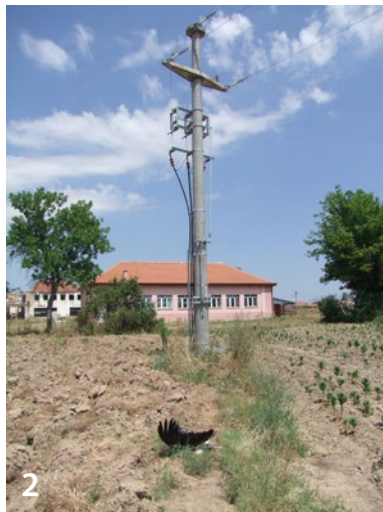
1 Endmasten mit Stützisolatoren aus Komposit 10-20 kV (Trap ID 358) – Totfund Weißstorch C. ciconia – 1 Terminal pole whit uninsulated jumper cables mounted on composite pin insulators 10-20 kV (Trap ID 358) – found dead White stork C. ciconia
