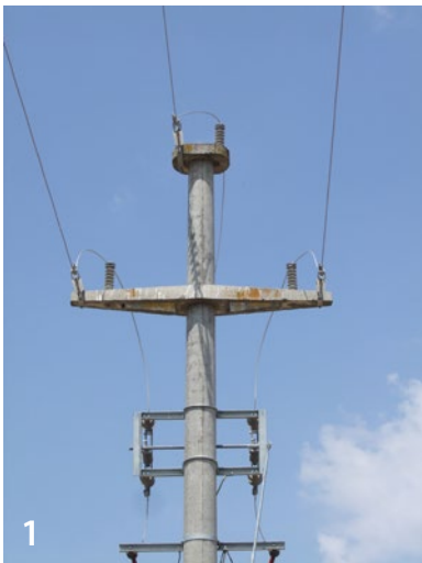
1 Endmasten mit Stützisolatoren aus Komposit 10-20 kV (Trap ID 358) – Totfund Weißstorch C. ciconia – 1 Terminal pole whit uninsulated jumper cables mounted on composite pin insulators 10-20 kV (Trap ID 358) – found dead White stork C. ciconia
