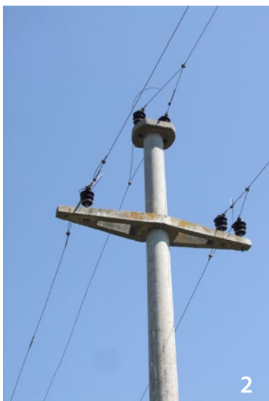
1 Tragmasten mit Stützisolatoren aus Komposit 10-20 kV (Sarandinovo ID95) – Totfund Adlerbussard B. rufinus – 1 Support pole with composite pin insulators 10-20 kV (Sarandinovo ID95) – found dead Long-tailed Buzzard B. rufinus
