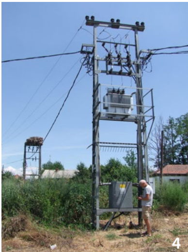
4 Transformatormasten aus Stahlgitter mit Stützisolatoren 10-20 kV (Optichari ID451) – Totfund Elster P. pica – 4 Transformer pole made of steel mesh with pin insulators, 10-20 kV (Optichari ID451) – found dead Magpie P. pica
