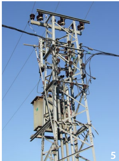
4 Transformatormasten aus Stahlgitter mit Stützisolatoren 10-20 kV (Optichari ID451) – Totfund Elster P. pica – 4 Transformer pole made of steel mesh with pin insulators, 10-20 kV (Optichari ID451) – found dead Magpie P. pica
