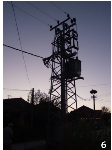
4 Transformatormasten aus Stahlgitter mit Stützisolatoren 10-20 kV (Optichari ID451) – Totfund Elster P. pica – 4 Transformer pole made of steel mesh with pin insulators, 10-20 kV (Optichari ID451) – found dead Magpie P. pica
