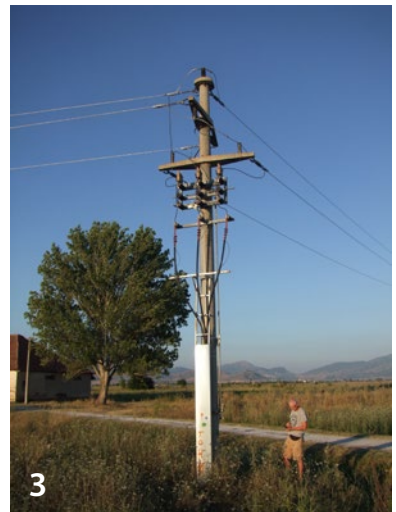
1 Endmasten mit Stützisolatoren aus Komposit 10-20 kV (Trap ID 358) – Totfund Weißstorch C. ciconia – 1 Terminal pole whit uninsulated jumper cables mounted on composite pin insulators 10-20 kV (Trap ID 358) – found dead White stork C. ciconia
