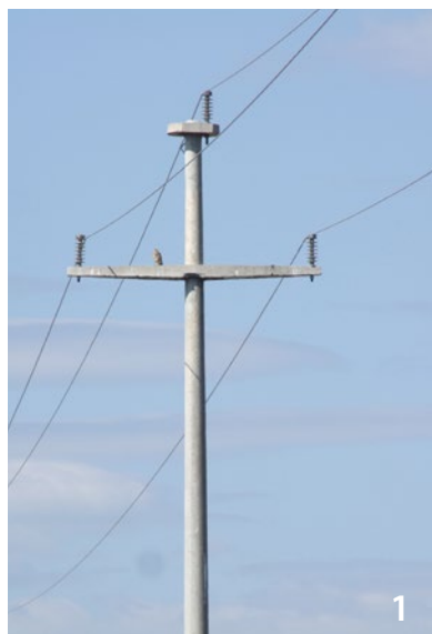
1 Tragmasten mit Stützisolatoren aus Komposit 10-20 kV (Sarandinovo ID95) – Totfund Adlerbussard B. rufinus – 1 Support pole with composite pin insulators 10-20 kV (Sarandinovo ID95) – found dead Long-tailed Buzzard B. rufinus
